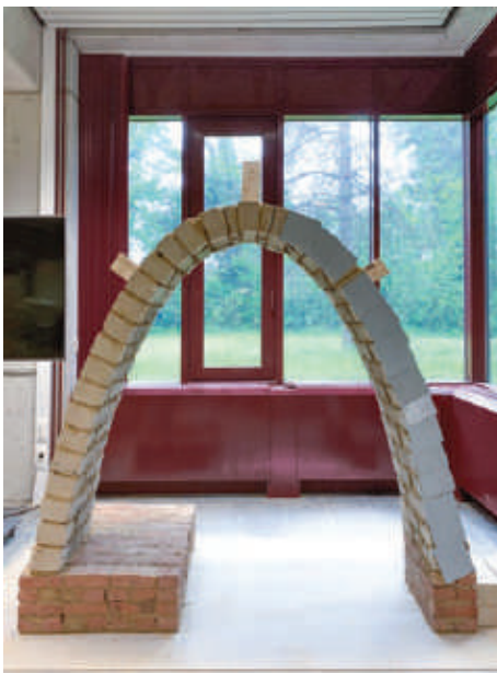
Figure 1 : Mock-ups with earth block masonry, designed and built by 3rd bachelor students in the Design&Build studio [Photo: Frank Vanden Ecker]
